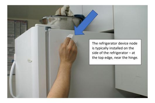
Clean the back of the device node with the wet wipe.
